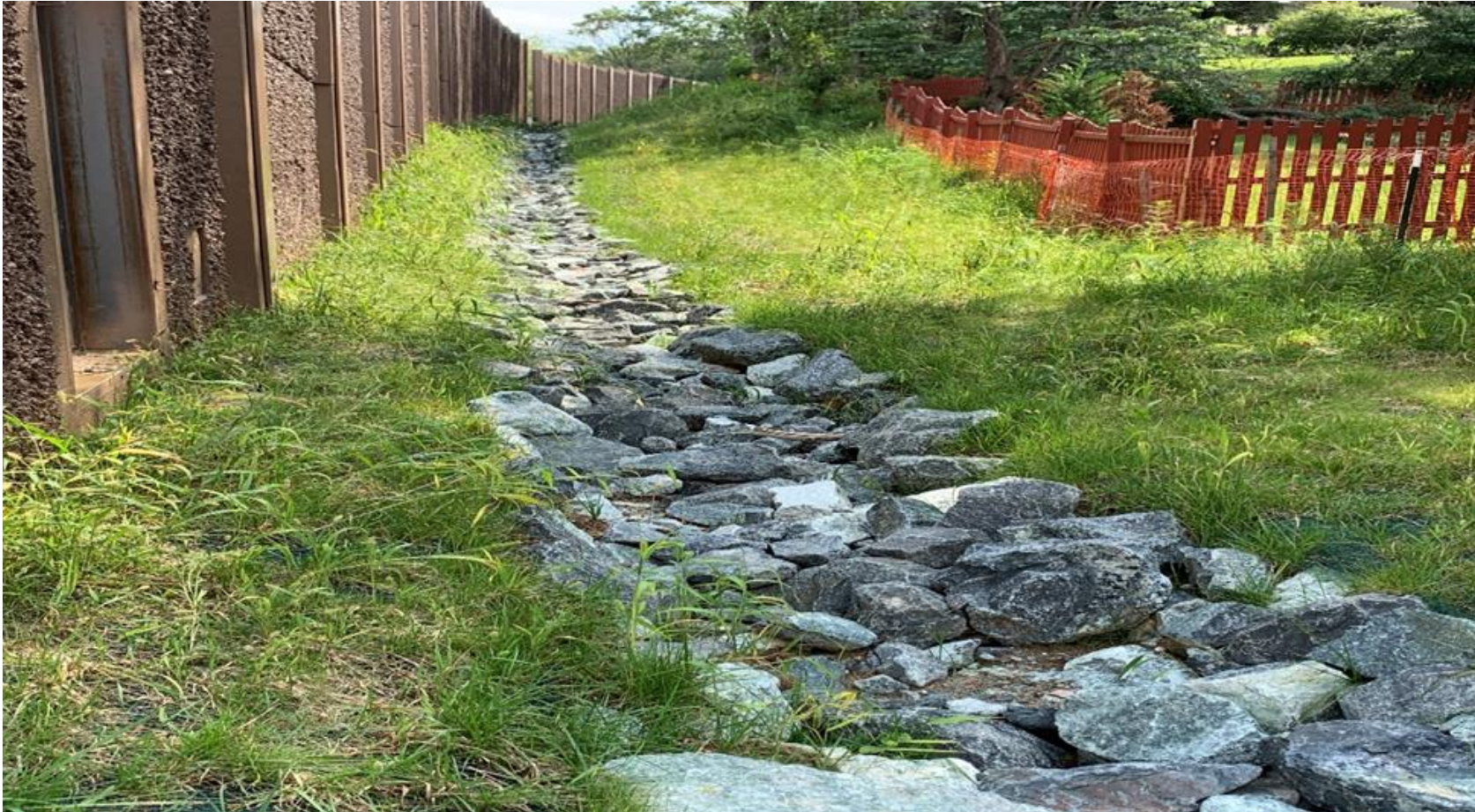
Completed Grading and Riprap Ditch Behind the Noisewall
